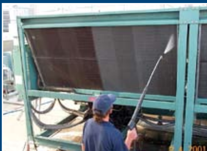
Pre treatment of condenser prior to the coating process.
