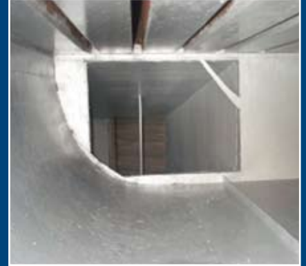
The process of entrusting, cleaning, primer treatment and finally the chemical resistant top coating.
